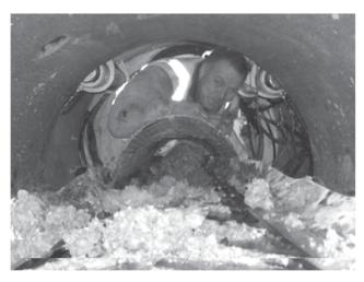
The picture above shows a conveyor belt removing the chalk dug out by the tunnelling machine on Shetland Road.
